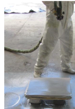
Fig. 2. Stages of the protection layers fabrication. Pulverization of PUC on support layers
